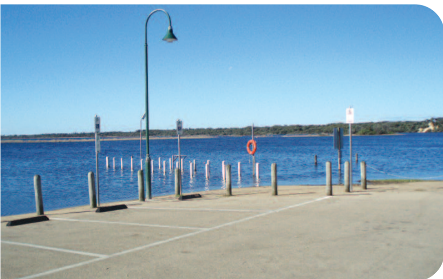
Flooded jetty at Lake Tyers, June 2014.
