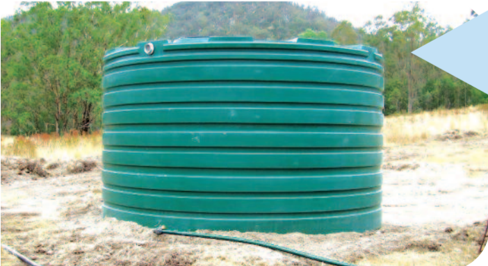
Tank for off-stream water system on the Wonnangatta River.
