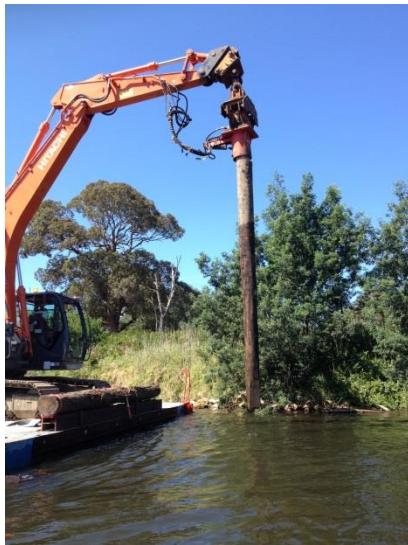
Wooden log fish habitats, tethered to a single pile near riverbanks
