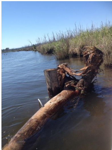
Wooden log fish habitats, tethered to a single pile near riverbanks
