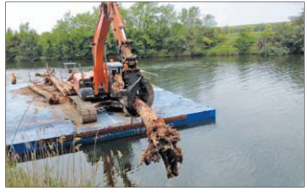
A Jarvis Norwood crew places a log in the Mitchell River. (PS)
