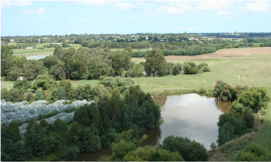
Works site, looking upstream.
