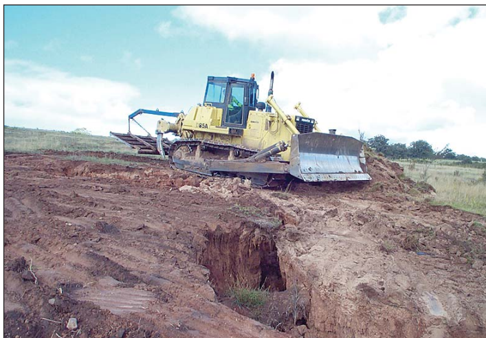
Repairing erosion at Glenaladale
