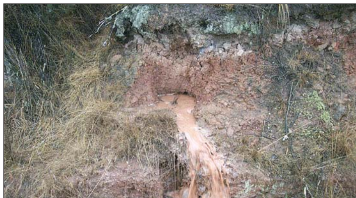
Tunnel erosion following rain
