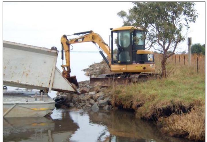
Placing rock on river bank
