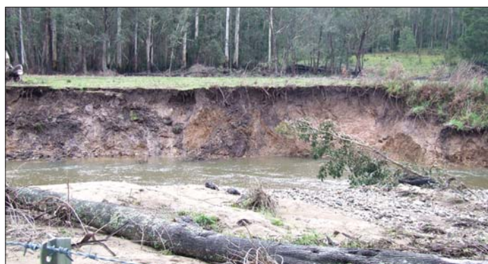
Vegetation loss increases the risk of flood damage
