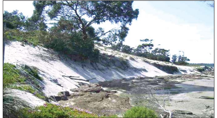
Round Head Project Before Works
