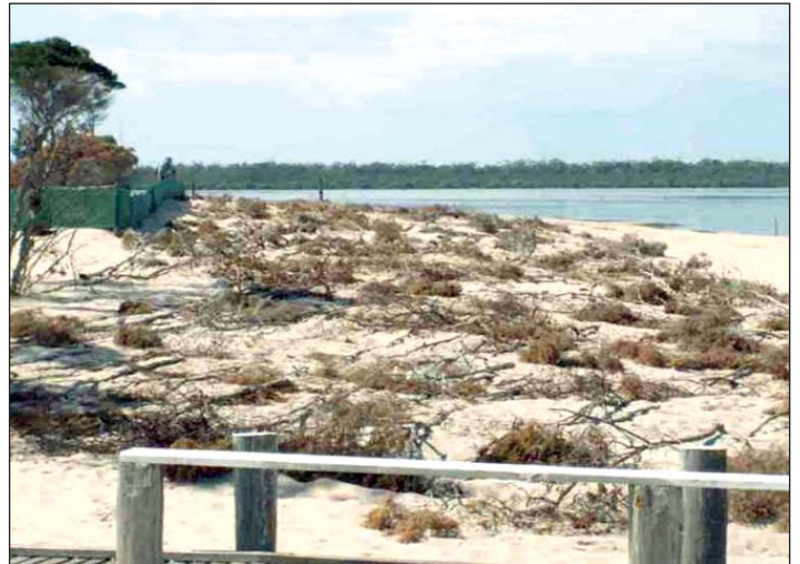
Round Head Project After Works
