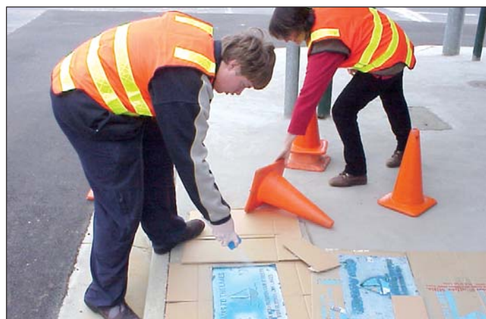
Spraypainting covers on stormwater pits
